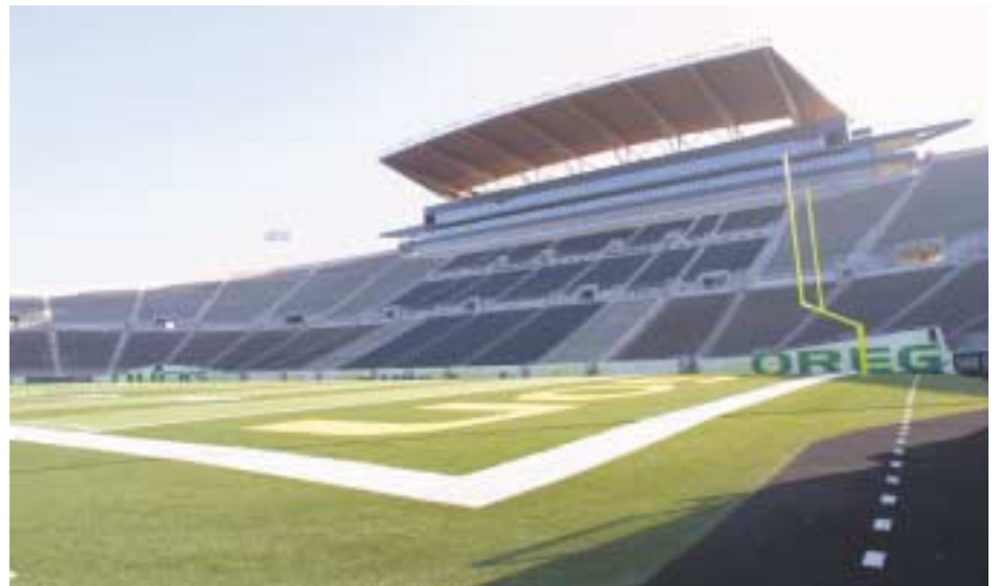
Autzen Stadium's new glulam roof structure cantilevers dramatically over enthusiastic (and now dry) Duck fans.
