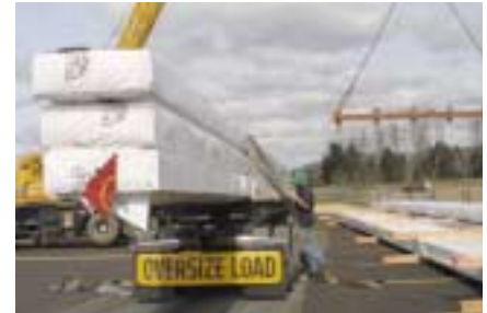
More than 430,000 board feet of Douglas-fir glulam was used in the project.
